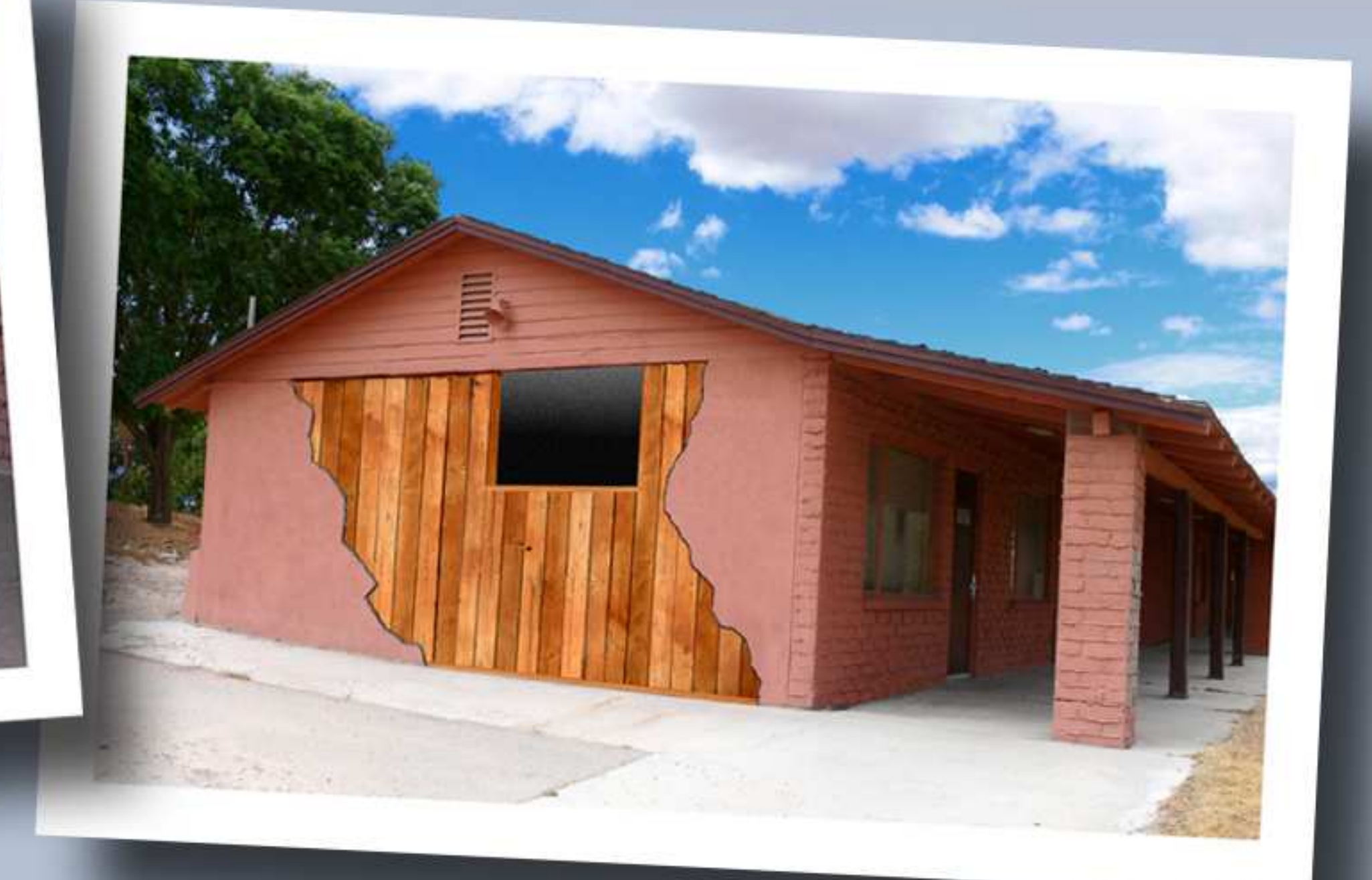
Cut away view of the railroad ties behind the stucco
