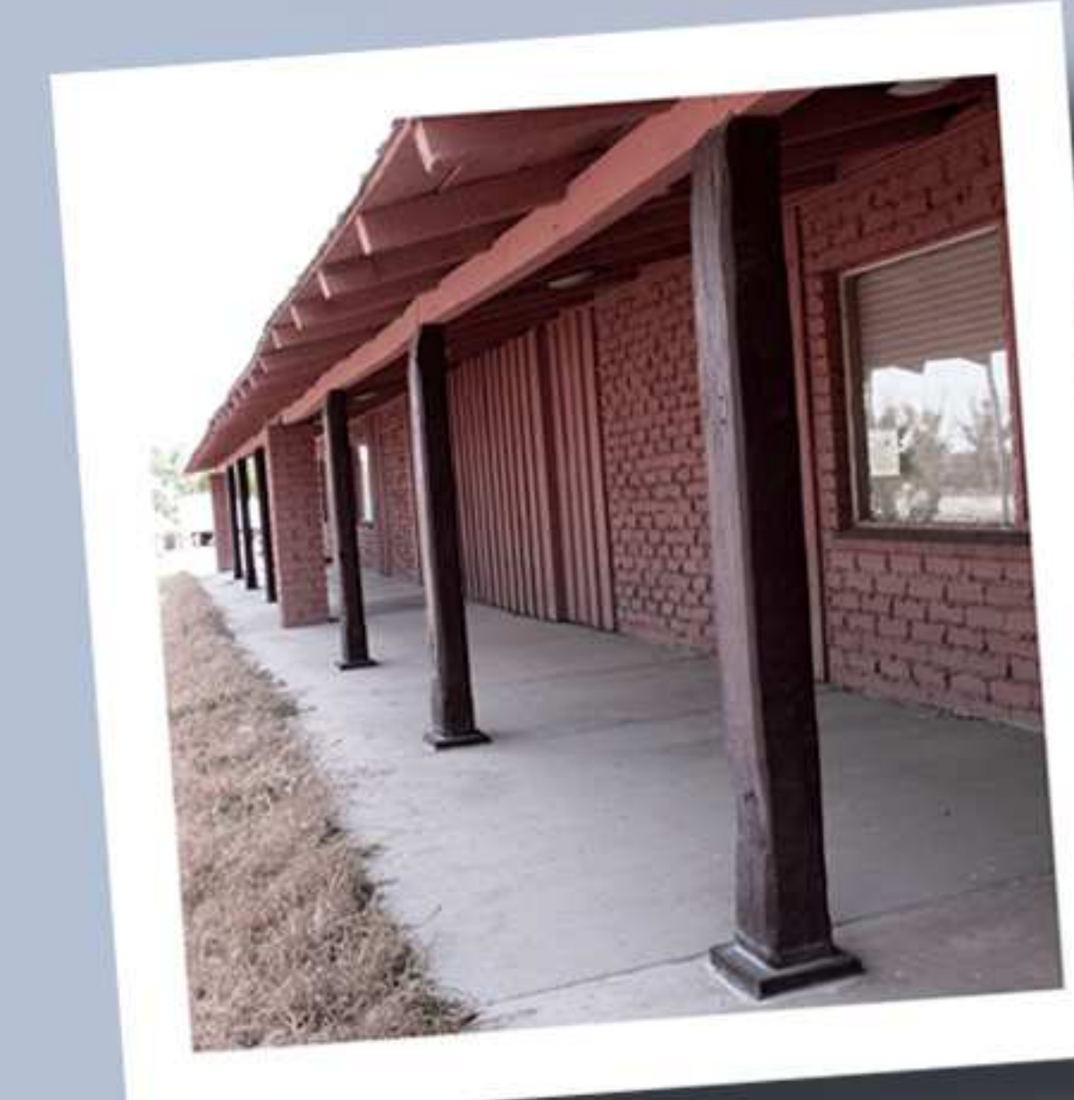
Railroad tie columns
